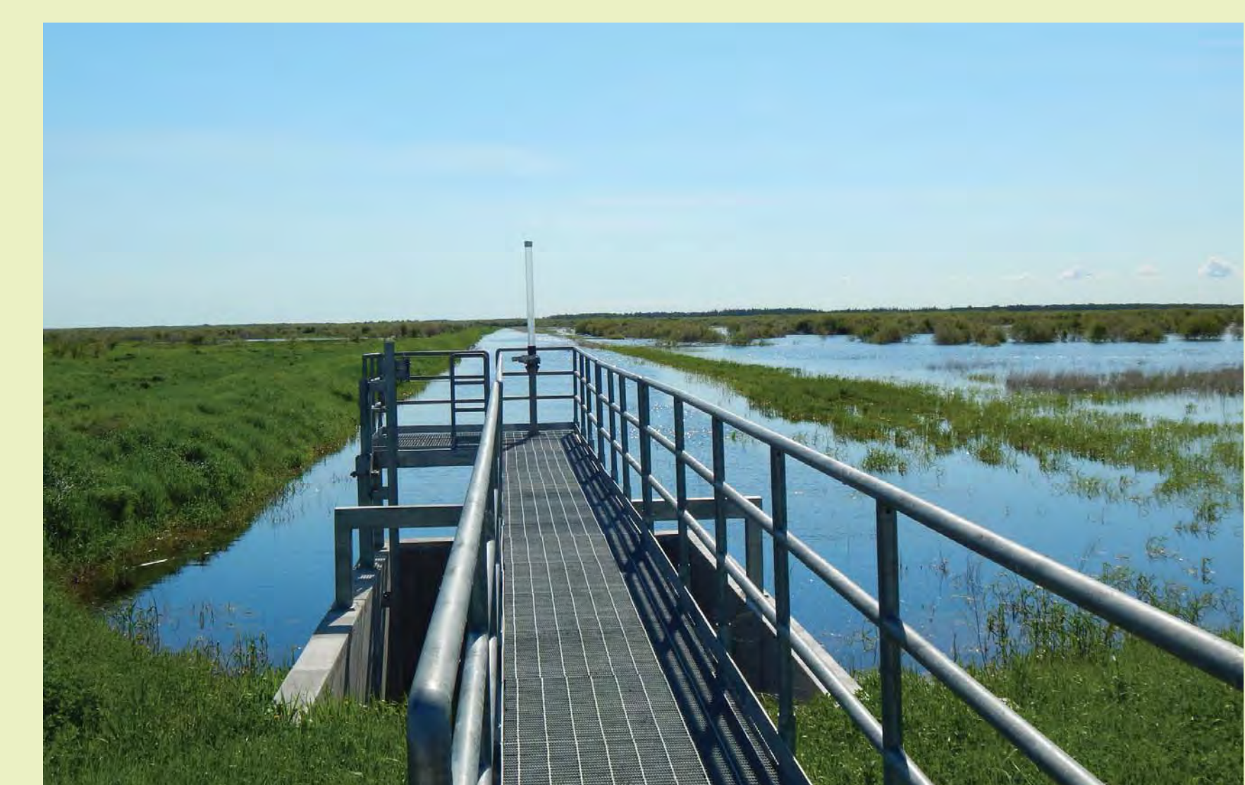
Norland impoundment "catwalk" over outlet structure, Photo: Tracy Halstengard
